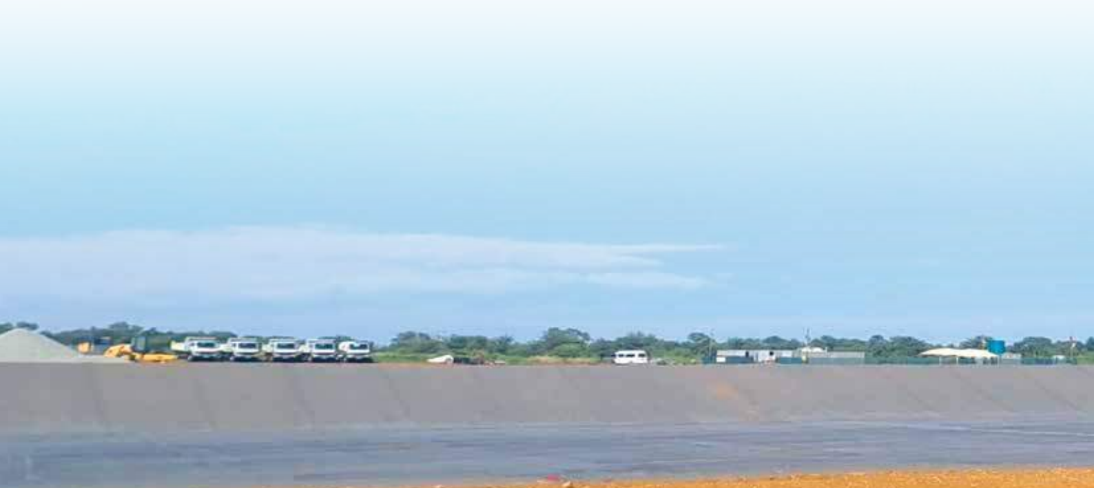
A new landfill cell lined with a membrane to prevent contaminated leachate from the landfill from contaminating the soil and groundwater, under construction at the Felophepa municipal landfill site in Potchefstroom, North West.
