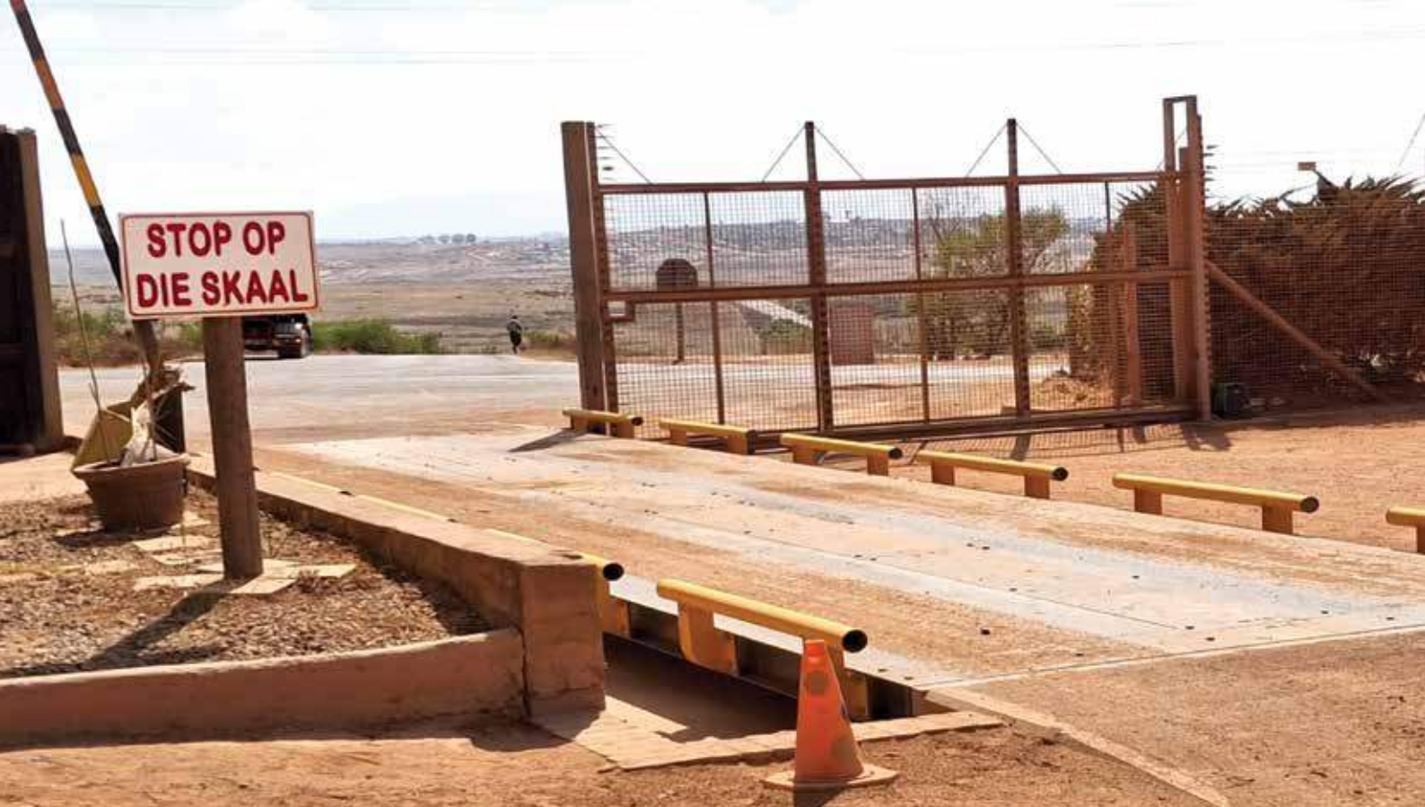
A working weighbridge and access control at the Malmesbury Highlands municipal landfill site in the Western Cape – one of only a few sites that can boast a 100% compliance rate in 2025.
