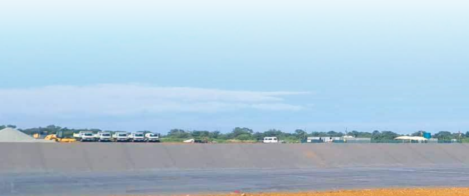
A new landfill cell lined with a membrane to prevent contaminated leachate from the landfill from contaminating the soil and groundwater, under construction at the Felophepa municipal landfill site in Potchefstroom, North West.
